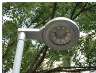
(改修後) LED 150W
